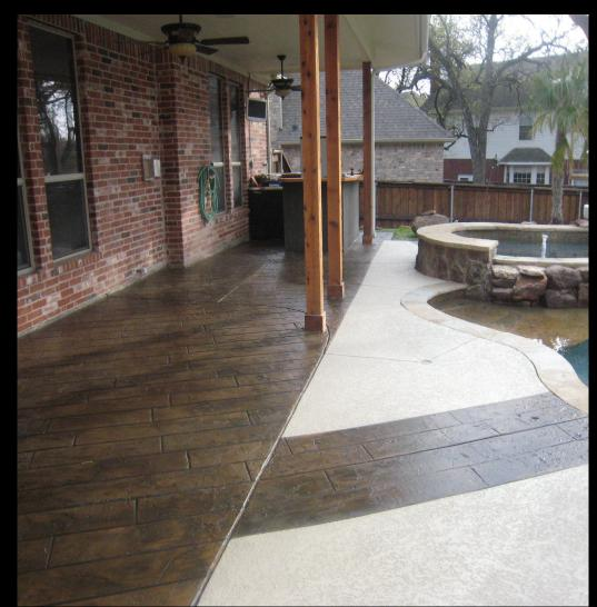
TUSCAN is a textured decorative concrete effect created by applying a thin overlay to an existing or new concrete surface. The Sundek artisan then creates a custom texture on the surface using their trowel and their experience, thus crafting a unique look resembling a deeper stamped concrete overlay.
