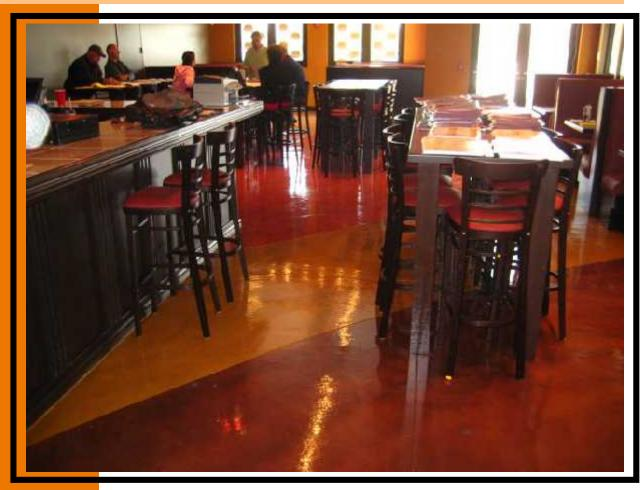
A water or solvent soluble Dye for concrete or overlay surfaces on interior projects
