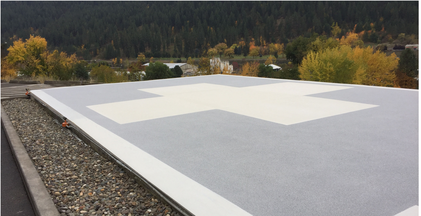
Photograph and installation by Knox Concrete
